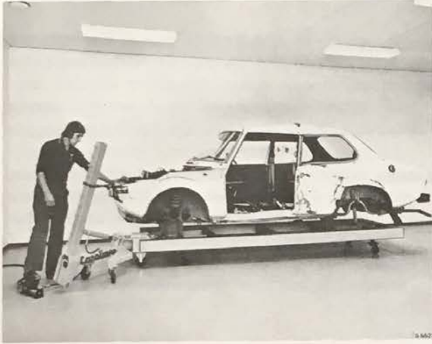
ALIGNMENT JIG, LATER VERSION
