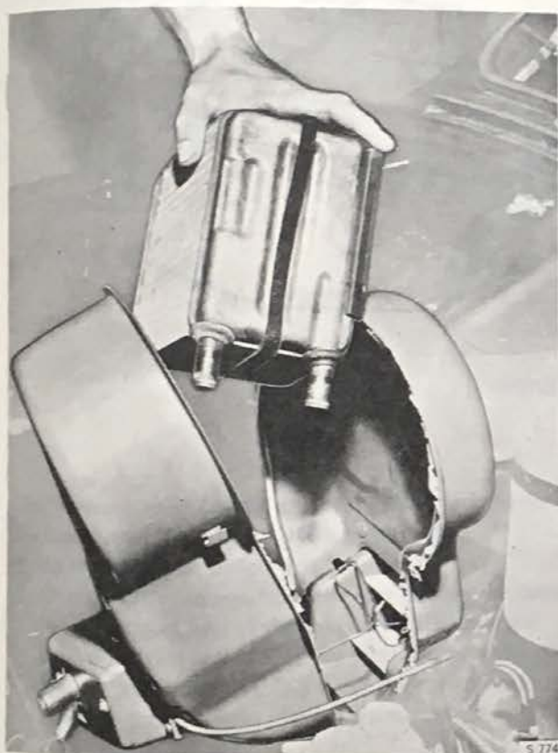
REMOVAL OF HEAT EXCHANGER
